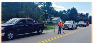
As part of a pavement management system, crack sealing can reduce pavement deterioration by restricting water penetration into underlying base and sub-base layers.
